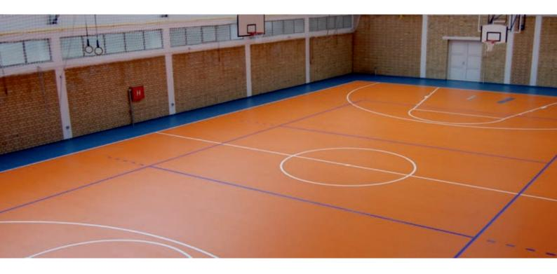
Our TEKNO Polyurethane based sports floor covering system is composed of the application of 4 different polyurethane components on top of the roll pad infrastructure that is produced out of the rand polyurethane and the recycle granulometric rubber mix that is 4-10 mm thick.
